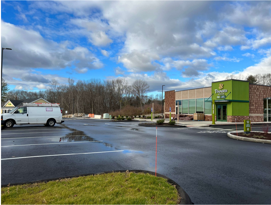
Existing Panera On Project Site
